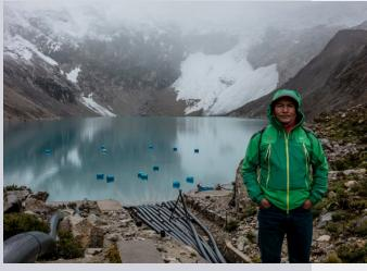
The glacier lake Palcacocha is currently equipped with a provisional pumping system, which is not sufficient to prevent a dangerous flood wave.
